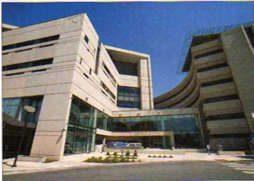
The view of Children's Hospital from the south has changed since the recent completion of its Clinical Expansion project.
